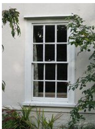
Example of a sash window
